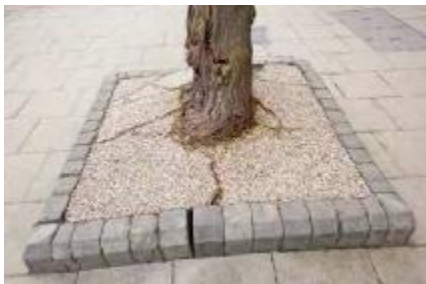
Cracked paving caused by growing roots
