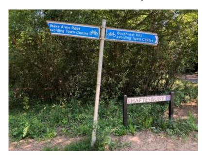
Sign pointing in the direction of Wakes Arms roundabout damaged beyond repair. To be replaced. I would suggest that the sign post be relocated to a position further from the junction than at present, as evidence would suggest the damage was caused by high-sided vehicles and proximity to the road.
