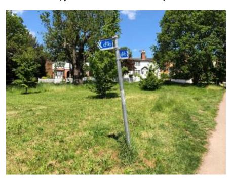
The sign post has been hit and is leaning. It was reinstated in July 2018 following a collision with a large vehicle (evidence in the shape of very wide indented tyre tracks), and because if this I would suggest that the sign post be relocated to a position further from the junction than at present, to give added protection.
